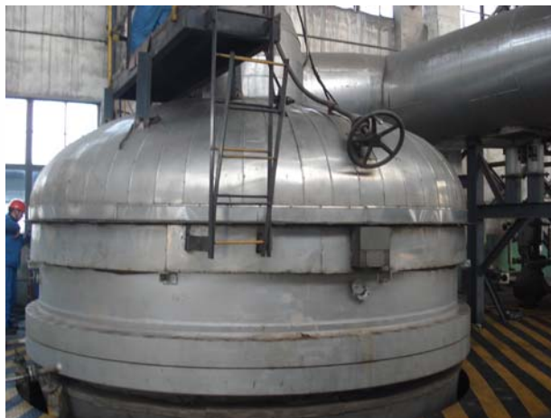
Figure 2. The ammonia burner with the installed de-N 2 O catalyst Figure 3. The existing ammonia burner at the plant
